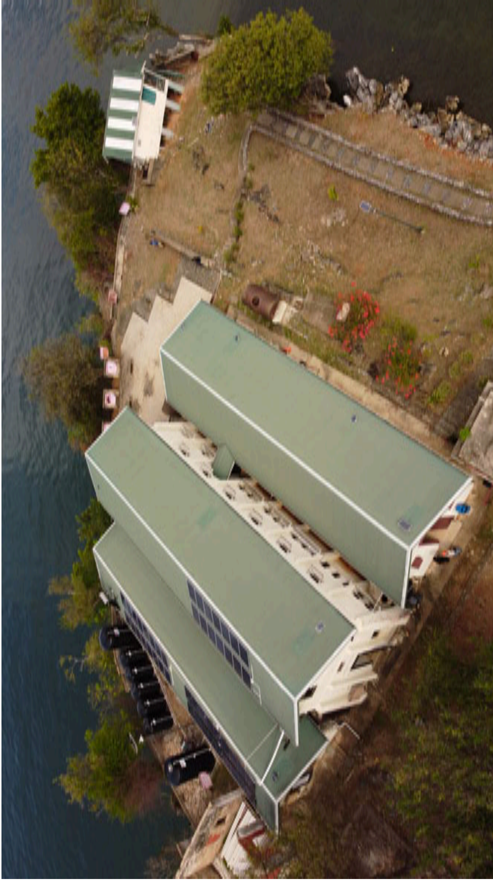
Drone photo of the west end of the island, showing the three main buildings and Butler cottage. An outdoor interpretive area is at the far end of the island, and the rugged terrain and trails are visible near the edge on the right.
